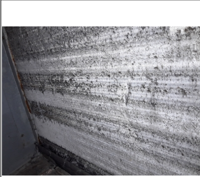
Evaporator coil needs cleaning
