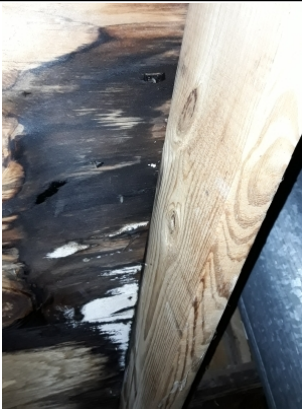
Wet roof decking above bonus room need to repair roof leak
