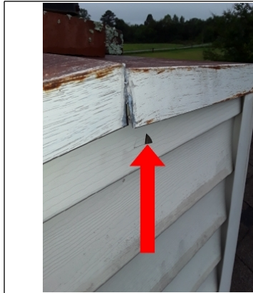
Hole in vinyl needs to be filled on chimney
