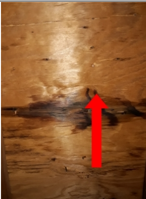
Wet roof decking above master bedroom need to repair roof leak
