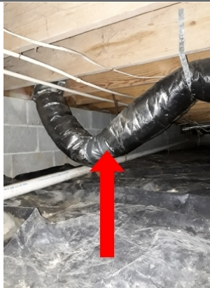
Flexduct needs to run as straight as possible for maximum air flow. Needs to be replaced
