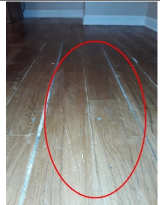
Floor is bowed and has gaps in wood looks like it has been wet before
