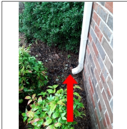
Down spout on front left hand side needs to be extended
