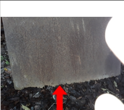
Crawl space door is rusted and missing metal at bottom needs to be replaced
