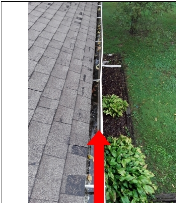
Gutter on back left side needs to be cleaned and aloped so it will drain
