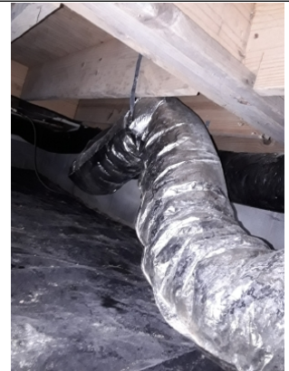
Flexduct needs to be straightened
