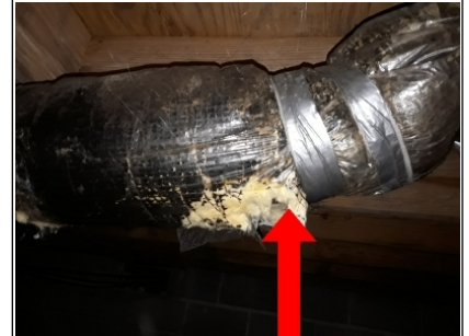
Flex duct needs to be replaced or repaired
