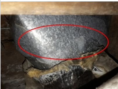
Hvac duct boot missing insulation
