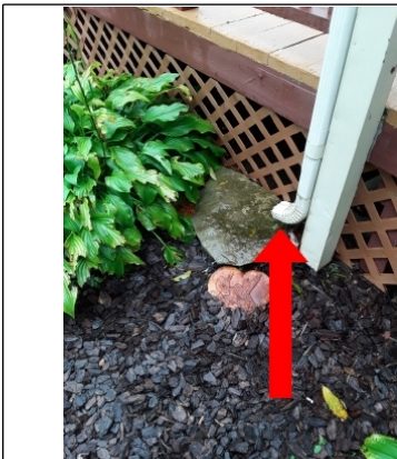
Down spout at pool deck needs to be extended
