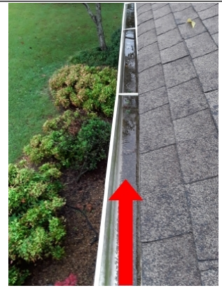
Gutter need to be sloped so it will drain
