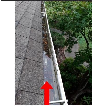
Gutter on right front of house needs to sloped so it will drain properly.
