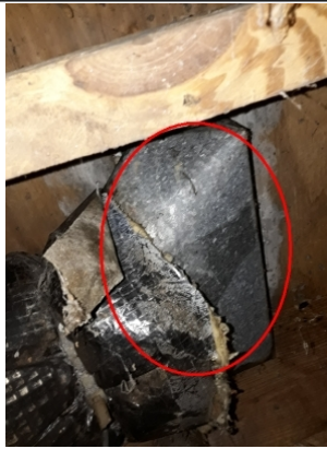
All Hvac duct boots need to be insulated
